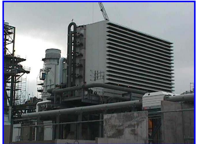
*Turnkey installation by TAS of a set of chiller coils in a GE 7FA / Donaldson filter house in 2002.*
