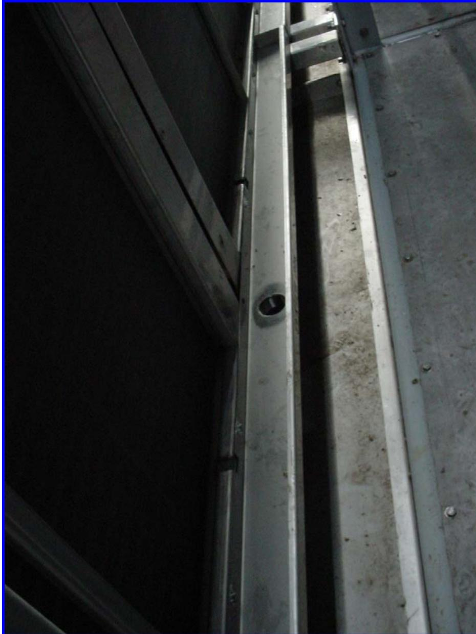
*Backside of Coil (looking down), showing part of drip pan. The hole in the center is for intermediate drains down to the Drain Sump*
