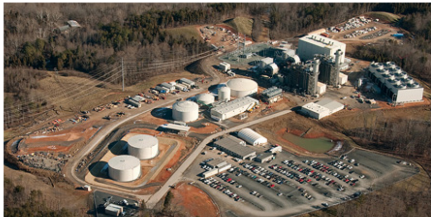
Bear Garden - 2 x GE 7FA - 60 MW Added - 7,800 chiller tons - 3.9 MG tank
