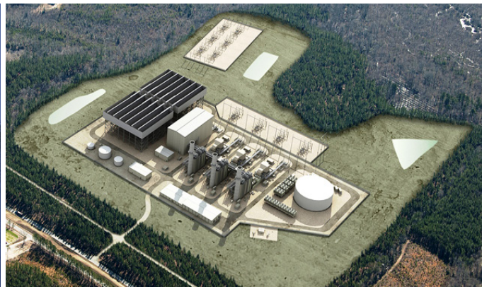
Brunswick County - 3 x MHI 501GAC - 123 MW Added - 29,300 chiller tons - 10.8 MG tank
