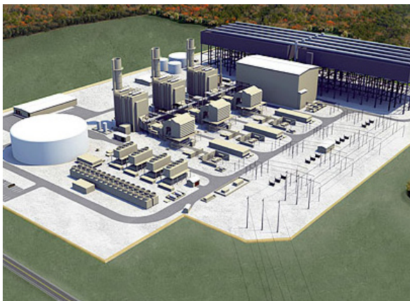
Greenville - 3 x MHI 501J - 132 MW Added - 29,600 chiller tons - 10.8 MG tank
