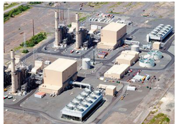
Fairless - 4 x GE 7FA - Retrofit - 115 MW Added - 11,200 chiller tons - 7.6 MG tank
