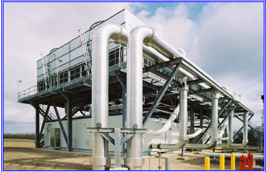
Two TAS F-50 chiller systems are shown installed with a common pipe rack, turning the two systems into a central chiller plant. The equipment in this picture represent the type of equipment discussed in the chiller system sections of this paper, providing sufficient capacity for two F-class gas turbines. The role of the chiller system is to produce cold water, which in turn is pumped to heat transfer coils at the GT filter house.
