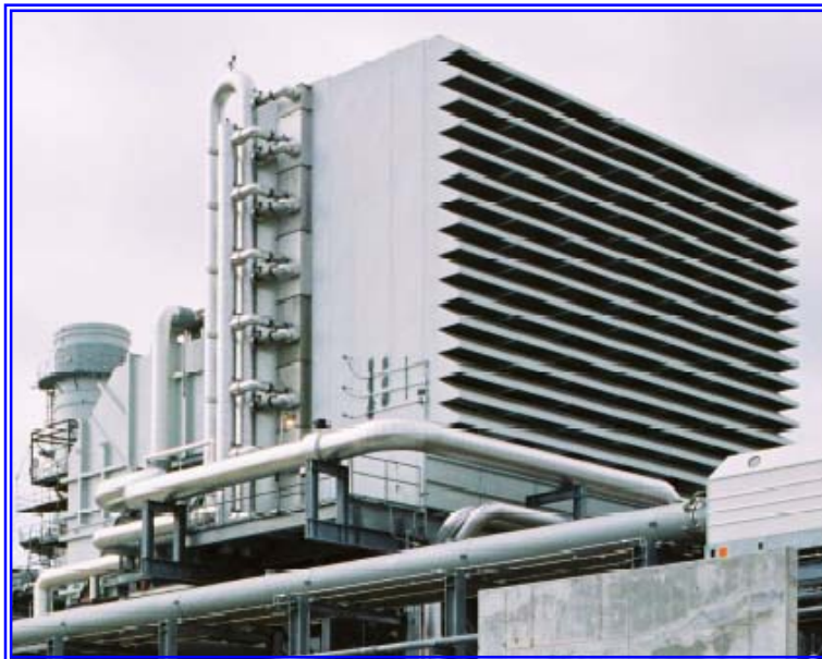
Two TAS F-50 chiller systems are shown installed with a common pipe rack, turning the two systems into a central chiller plant. The equipment in this picture represent the type of equipment discussed in the chiller system sections of this paper, providing sufficient capacity for two F-class gas turbines. The role of the chiller system is to produce cold water, which in turn is pumped to heat transfer coils at the GT filter house.
